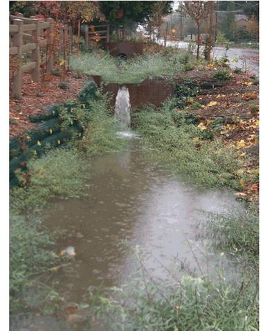
**Cascading bioretention cells in Seattle help treat and infiltrate stormwater from roads.**
