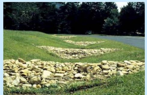
The rock check dams placed along this grassy swale help slow stormwater and prevent erosion in the swale (max. 6% slope).
