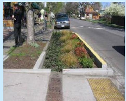
This roadside bioretention collects and treats roadway stormwater.
