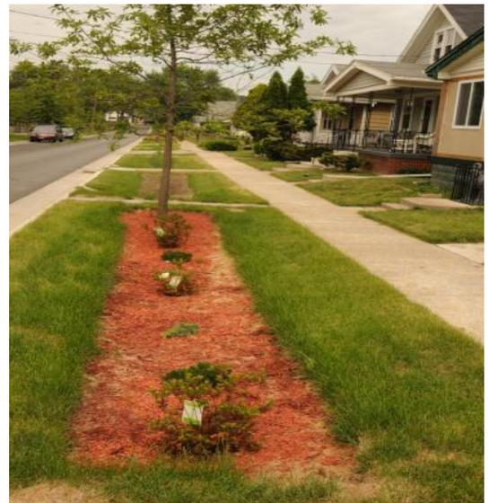
Roadway and sidewalk stormwater drain to this roadside bioretention system on Maywood Avenue in Toledo, Ohio.
