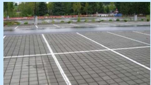
**This large parking lot helps to infiltrate stormwater through a permeable pavement system.**
