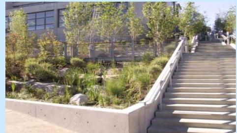
**Stormwater from a rooftop drains into this terraced bioretention facility.**
