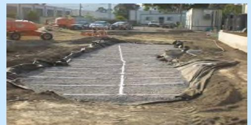
**This underdrain pipe system will help to drain the bioretention area above it.**
