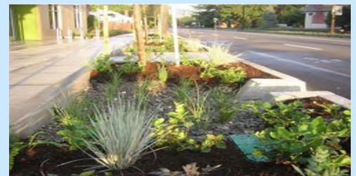
**When this bioretention planter box is full of stormwater, the extra water "backs up" into the street to drain into a storm inlet.**
