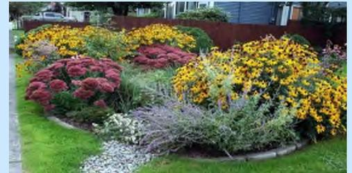
**A stone channel is used in this residential rain garden to direct overflowing stormwater to the street.**
